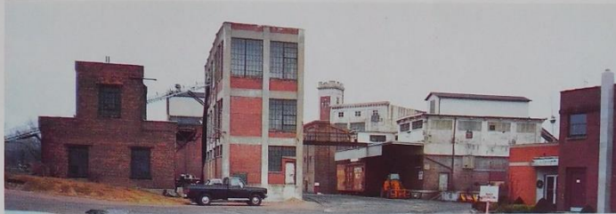
PNER 77 is out of commission (permanently) near the Carbon Sales plant. In the background is another view of the facility with the storage and loading building in the center of the photo. Modelers should note such details as the conveyor servicing the one-ton bag packaging building, the abandoned brick stack at right and the pile of wood pallets waiting for stacks of packaged culm coal.
