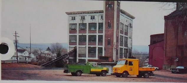
Carbon Sales in Miners Mills, Pa., has converted an abandoned flour mill into a culm coal packaging plant. This view features the building in which the 100-lb. sacks are packaged. Note the conveyor which carries coal from the truck dumping pit into the building. In the foreground are maintenance vehicles belonging to the Pocono Northeast Railway.
